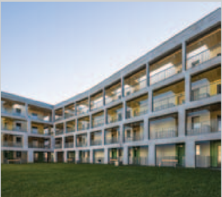
100 flats passive house, Budapest
