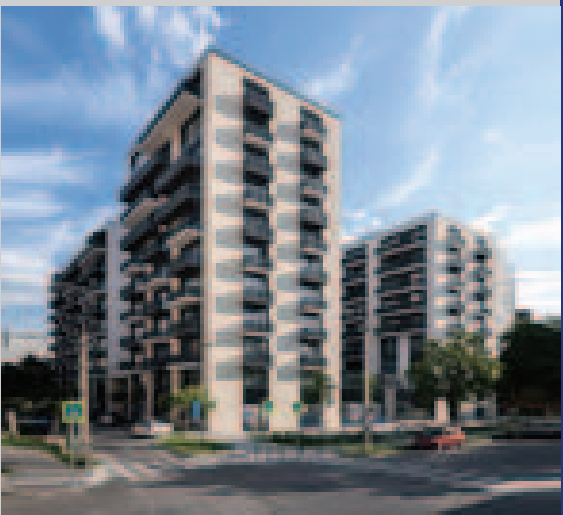
Flatco Apartment house
